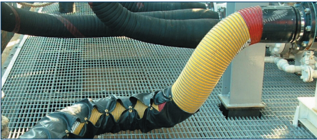
Figure 4. Non-conductive cover installed on the vapour hose.
